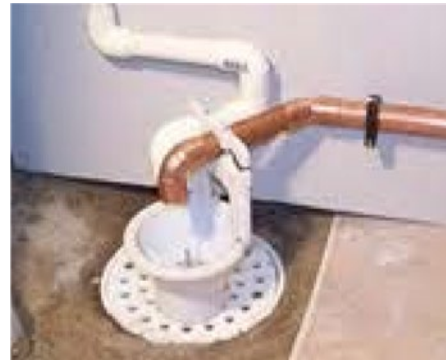
Drainage of the softener discharge line to a floor drain with an air gap
