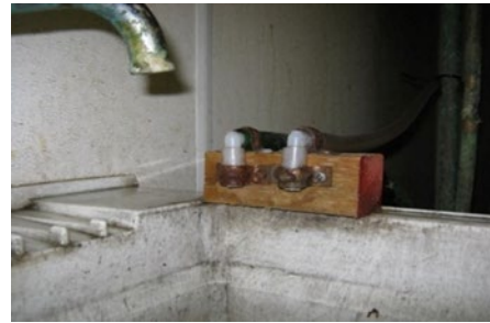
Placing the softener discharge drain line into a sink with an air gap
