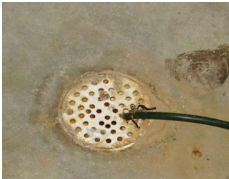
Drainage of the softener discharge line to a floor drain without an air gap
